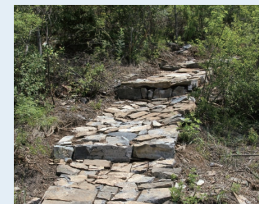
Green trail built as part of the project's ecotourism activities.
