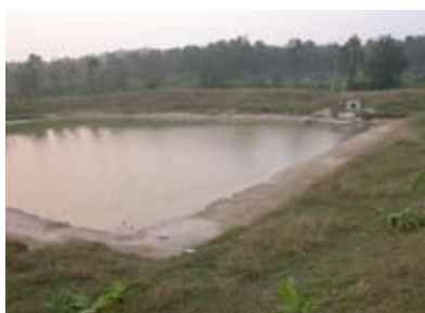
Protection of water sources
